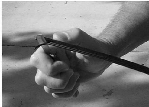
**Figure 1 – Cut the rib between the toning wire and cable.**
