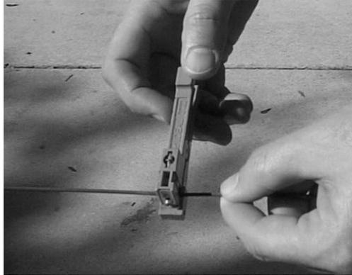
**Figure 8 – Score the buffer tube at the proper length.**
